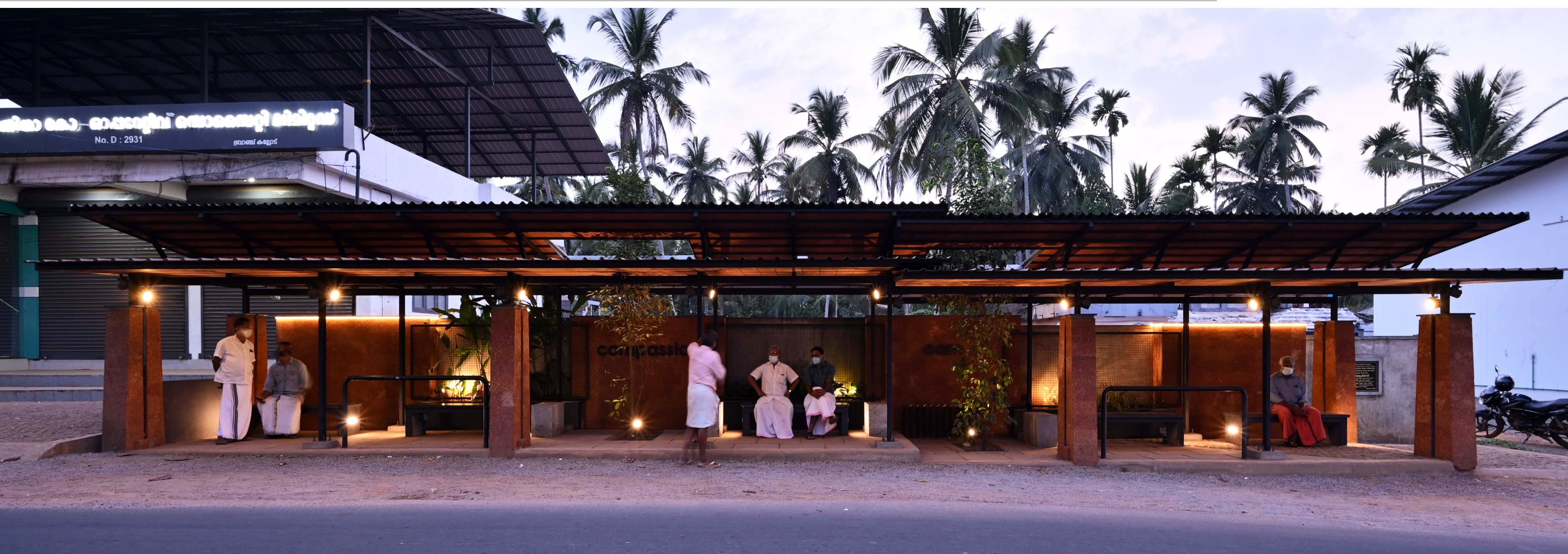
MATERIAL PALETTE AND BUILT FORM The warm palette of materials used include locally available laterite, stone, concrete for the benches, onduline sheet for the roof and terracotta ceiling tiles below. The scale is intimate and the built form merges with the setting.
